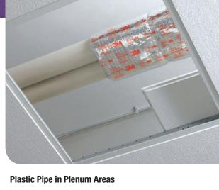
3M™ Fire Barrier Plenum Wrap 5A+ meets test criteria for use on plastic pipes located in plenum areas.
