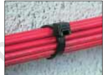
4. Install wires or cable.
