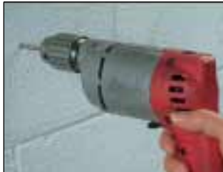
1. Drill hole using correct size bit.
