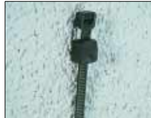
3. Place cable tie through mount.
