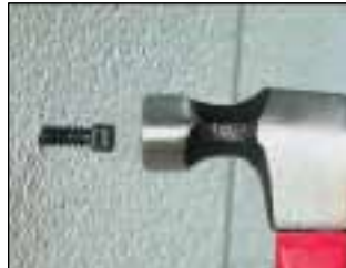
2. Hammer mount into hole.
